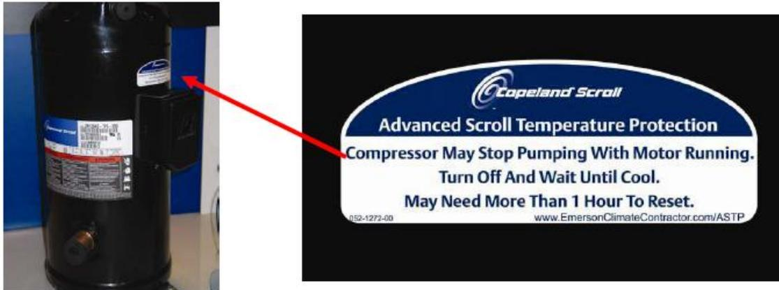
Figure 14: Advanced Scroll Temperature Protection (ASTP)
